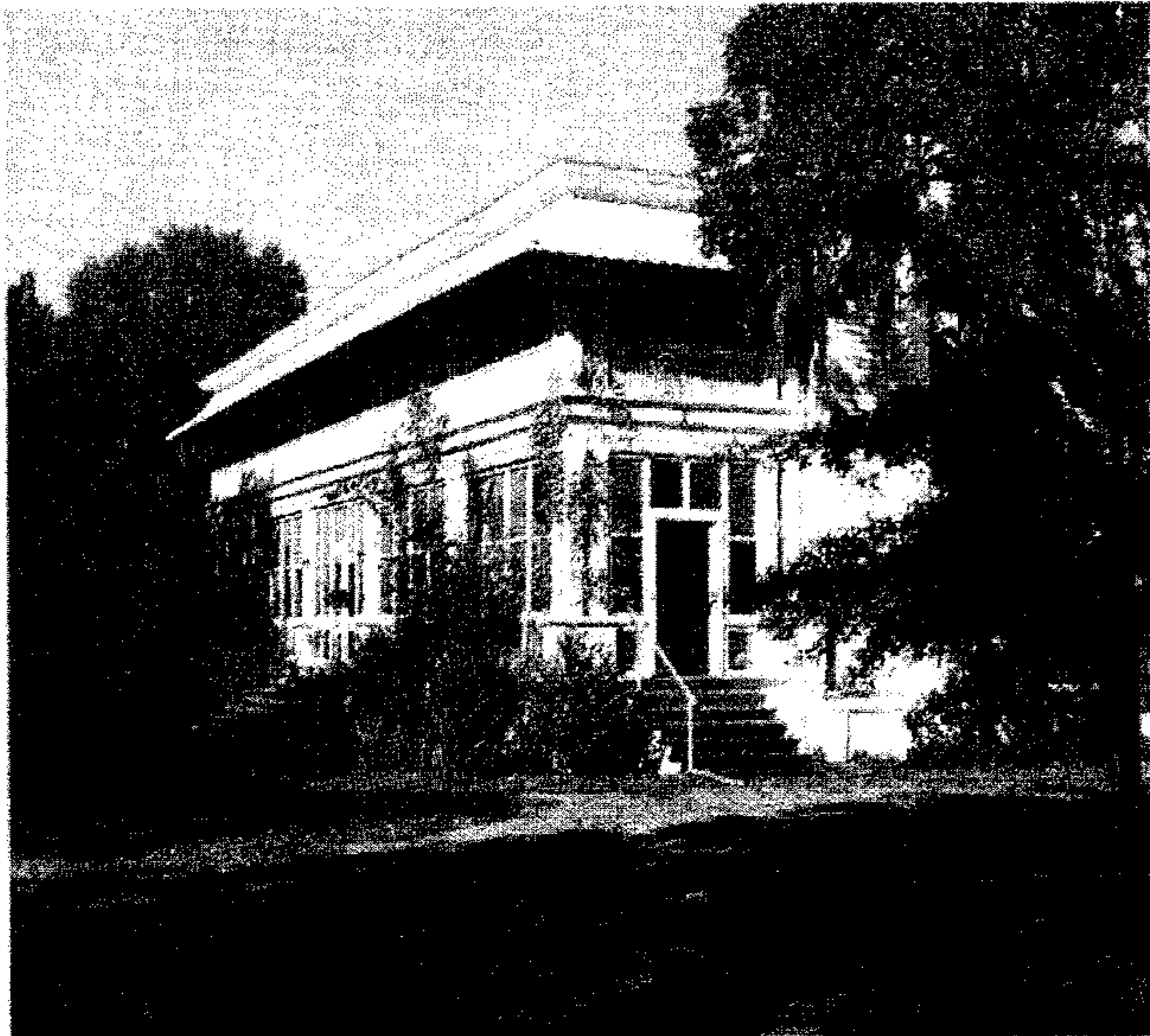
The historic base commander's residence on the former Charleston Naval Base is one of the base's three historic houses being restored by South Carolina STRONG.
